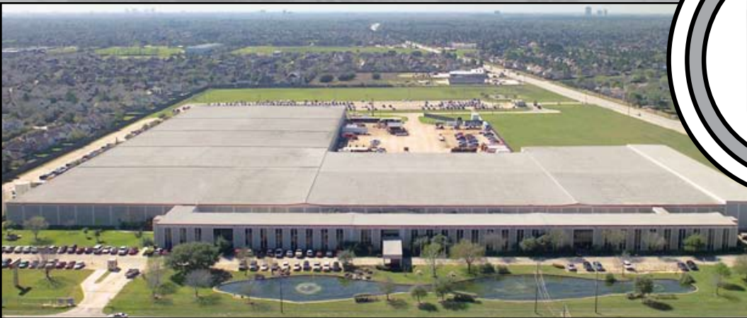
North American Headquarters & Manufacturing Facility (Houston, TX)
