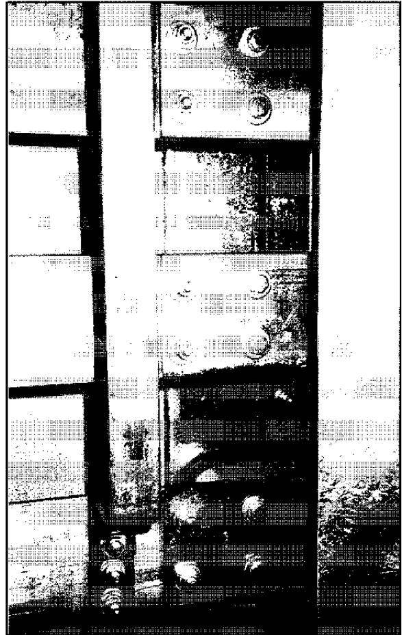
Fig. 28 Bus Splice Links
