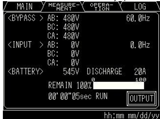
FIGURE 2.4.3 Values in Battery operation
