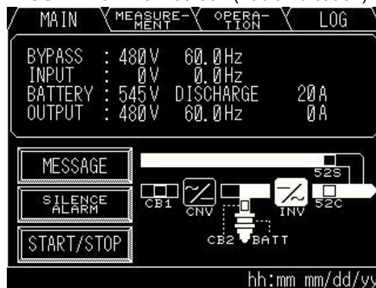
FIGURE 2.8 Main screen (Fault indication)
